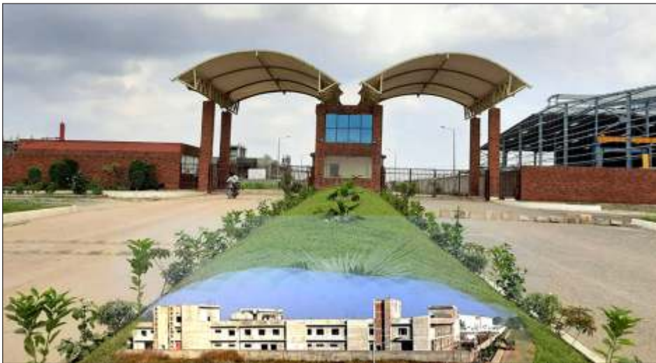
ELCINA ELECTRONICS MANUFACTURING CLUSTER, BHIWADI, RAJASTHAN, KHUSHKHERA
