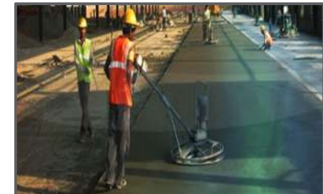
FLOOR REPAIR & RESTORAT
