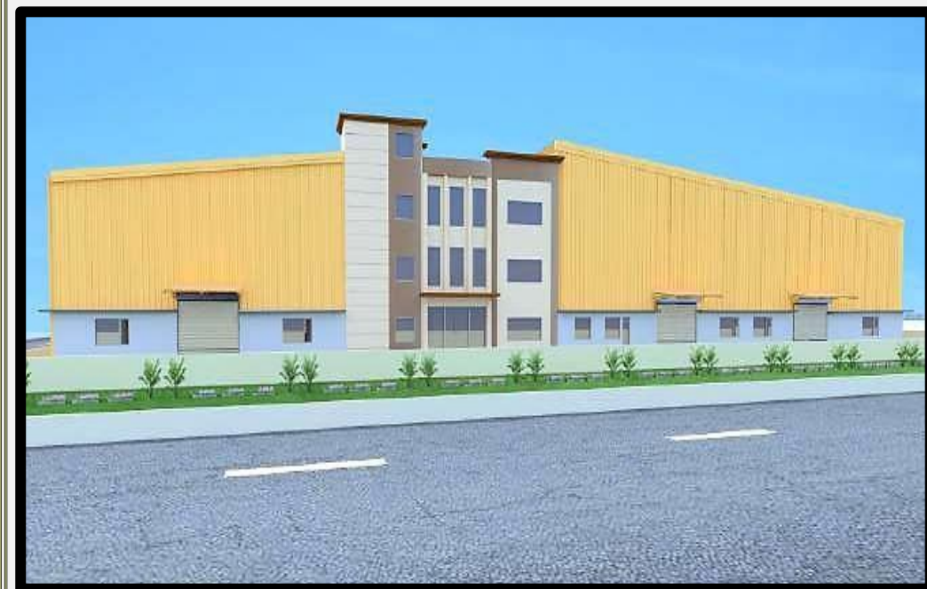
MALHOTRA CABLES PVT LTD, KAHARANI, BHIWADI
