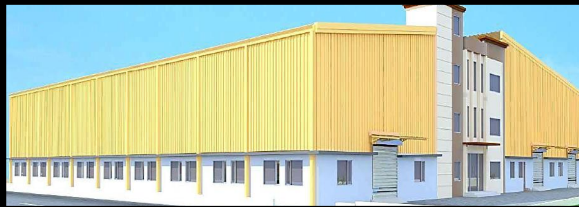
MALHOTRA CABLES PVT LTD, KAHARANI, BHIWADI
