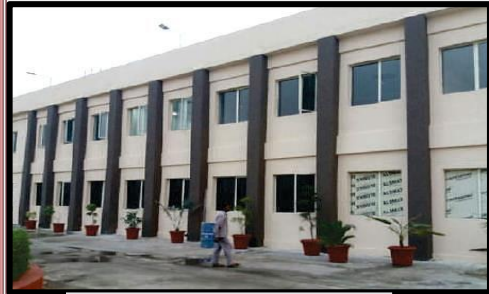
MAHLOTRA CABLES (Unit 2)
