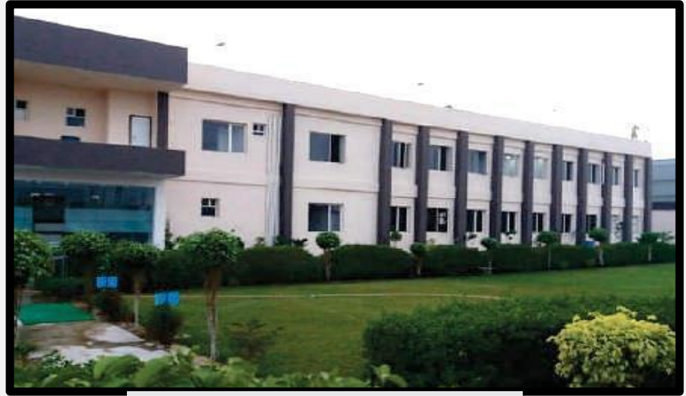
MAHLOTRA CABLES (Unit 2)
